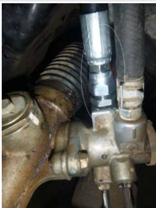
Image 4.2 Hydro boost to steering rack line
